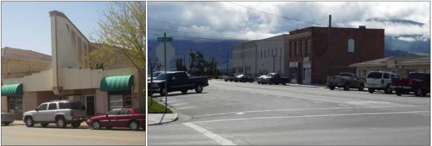
Left: Unoccupied theater building on Kidder Street. Right: Example of wide streets in the downtown area (looking west on Main Street at the Monterey Street intersection).
